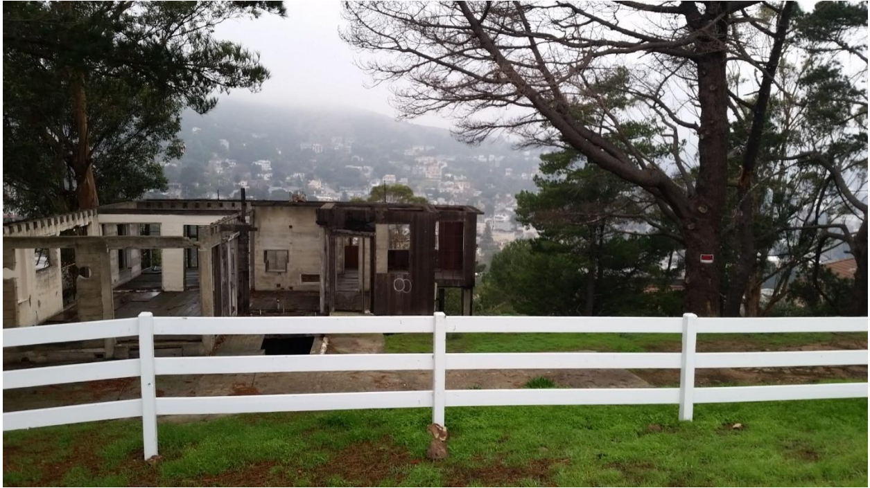
Photograph 1. Southernmost portion of the project site. (Standing east of the project site - offsite - facing west)
