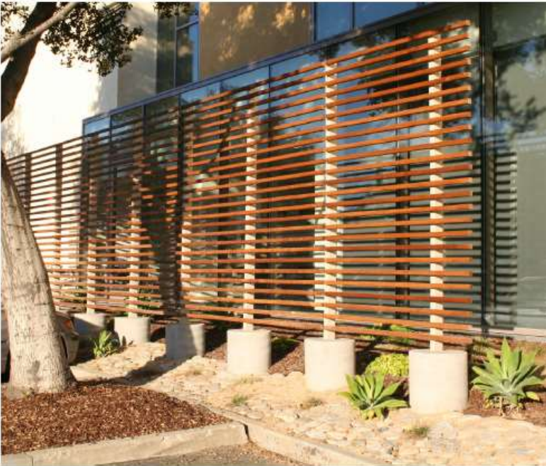
Subtle, well-designed screens should be used to allow daylight to enter while providing privacy to occupants.
